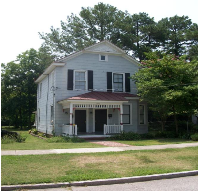
204 Hill Street -- $ 72,000 Physician's House – ca. 1920
